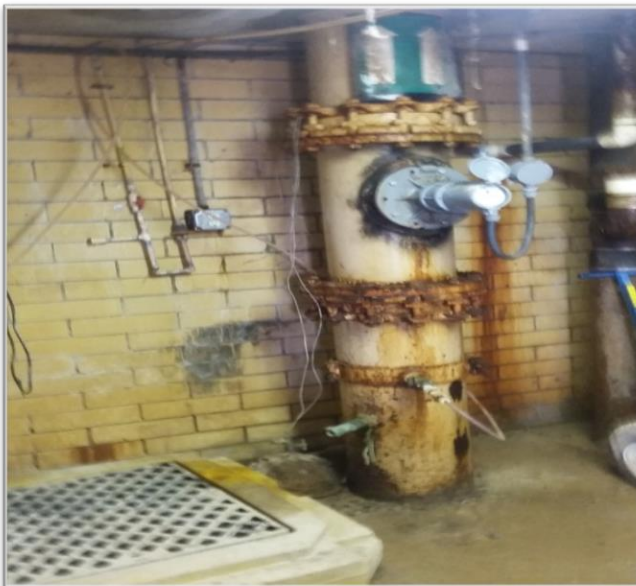
Mill Street Water Treatment Plant Condition
