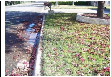
Examples of surfacing leaks.
