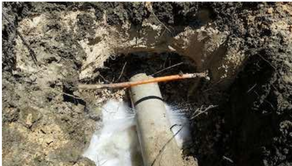
Example of Main Break Located on 8-inch AC Water Line
